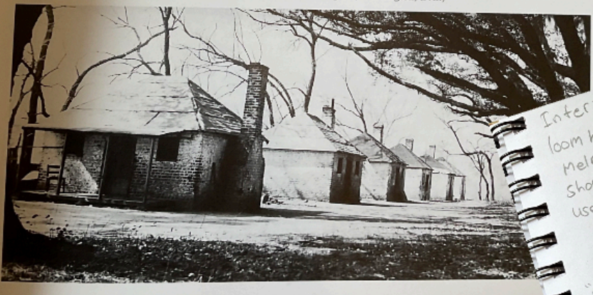
6. Whitewashed brick slave cabins from The Hermitage, Chatham County, Georgia. (Historic American Building Survey, Photographic Collection, Library of Congress, Washington, D.C.)
