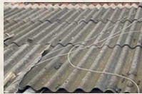
Corrugated fiber cement roofing
