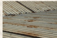
Corrugated metal roofing
